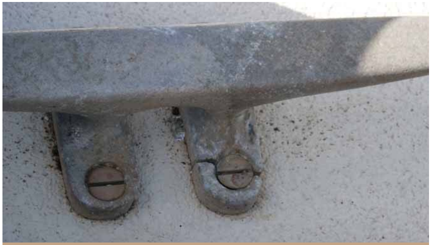
Stainless Steel Cleat Showing Corrosion Cracking
