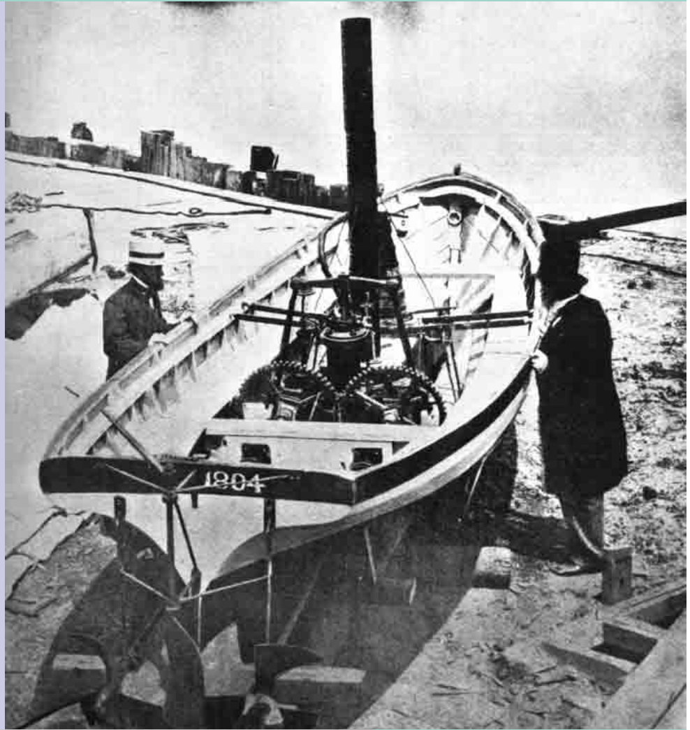
John Steven's 1804 steam-powered motorboat, with twin counter-rotating propellers.
